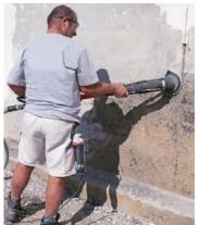
Grinding bitumen coating with PCD grinding disc
