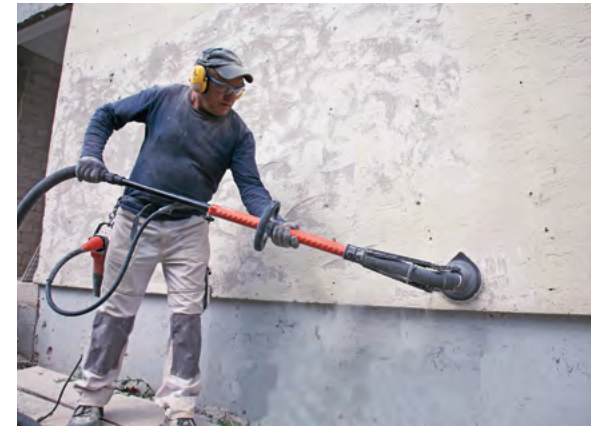
Removing old plaster and paints
