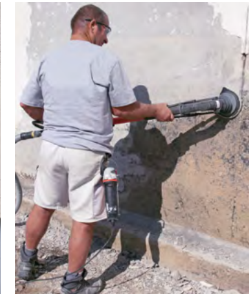
Grinding bitumen coating with PCD grinding disc
