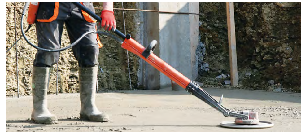
Levelling fresh concrete
