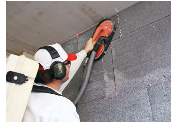
Grinding EIFS and ETICS boards
